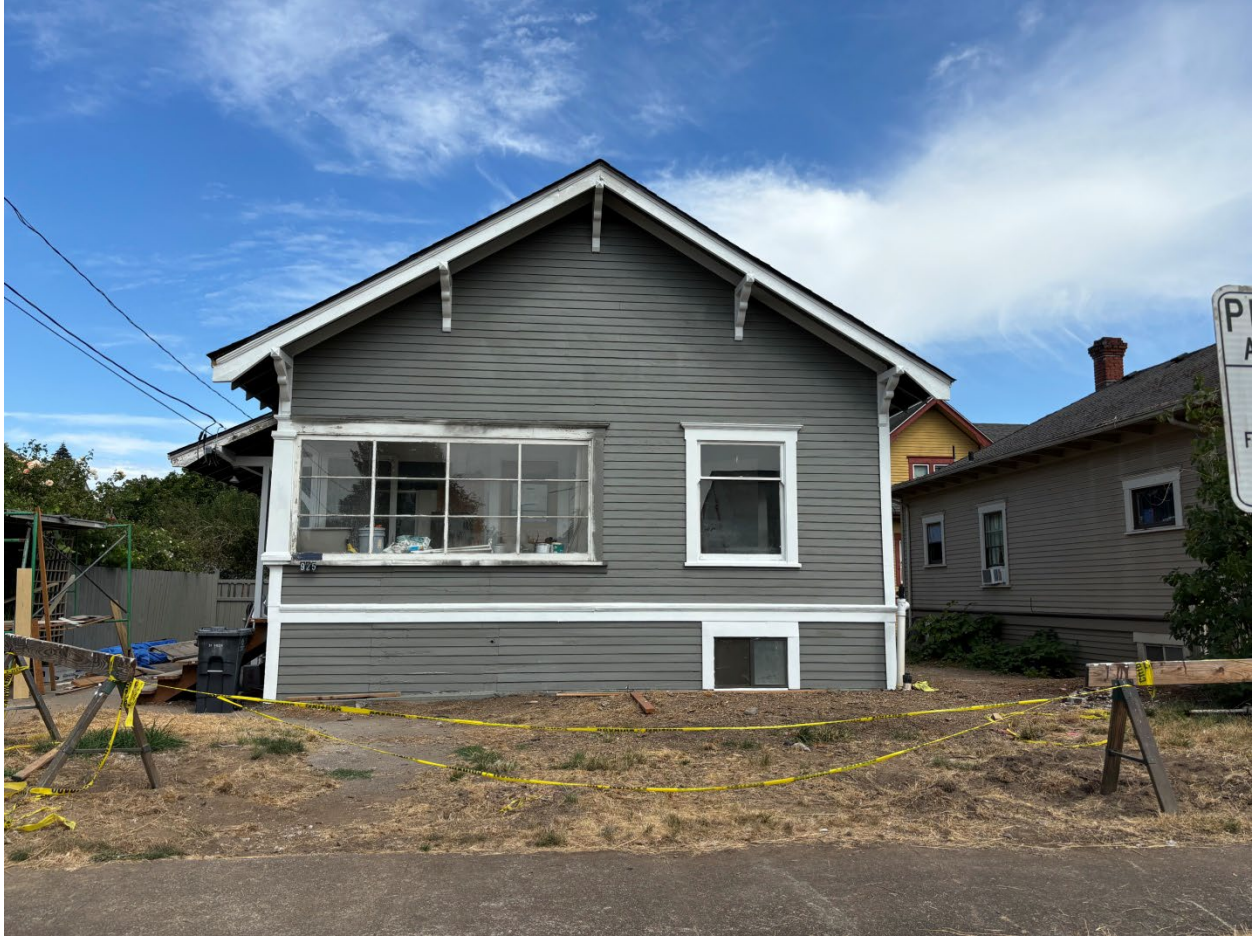
Painting in progress at 925 Walnut SW
