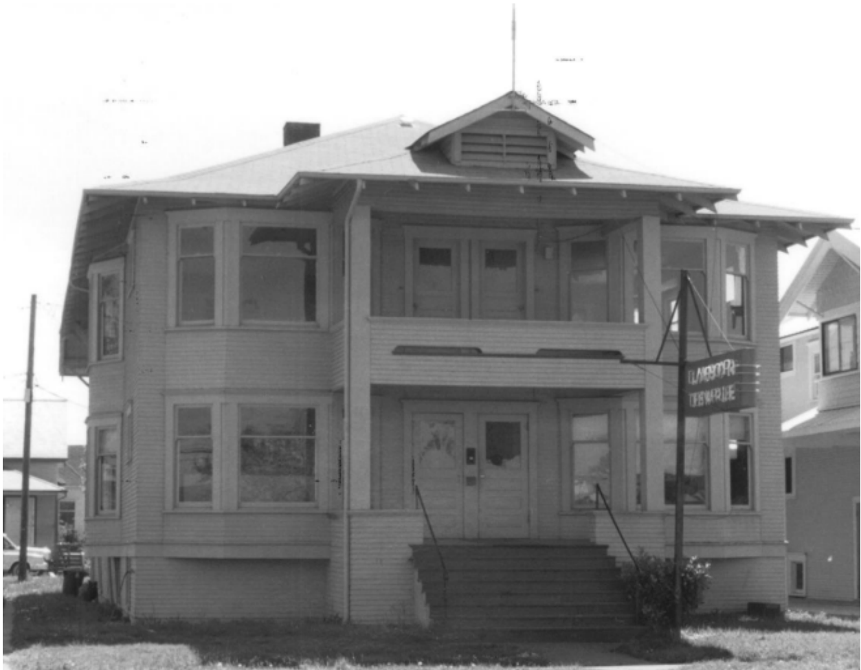
Figure 1: North Elevation, Historic Resource Form
