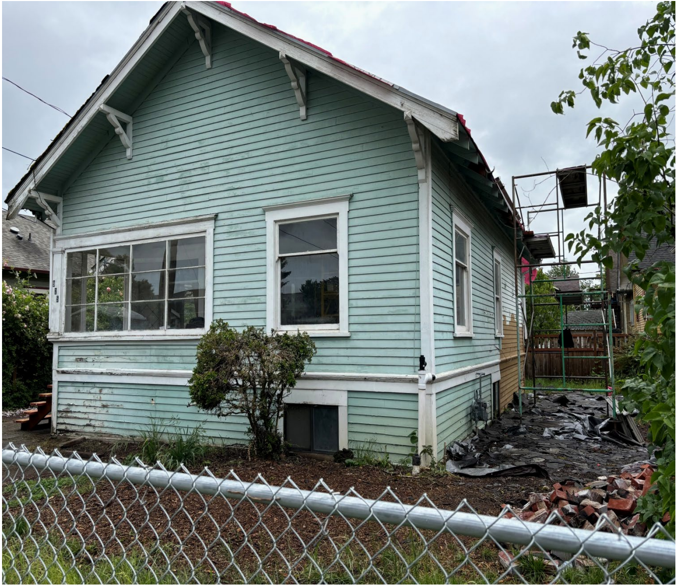
South side of house
