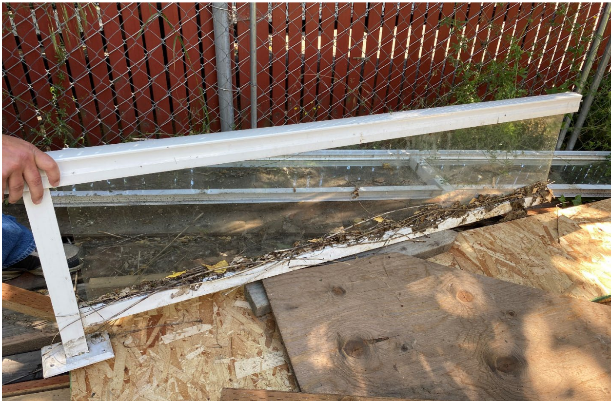
Figure 3: Approved Upper Front Porch Guardrail
