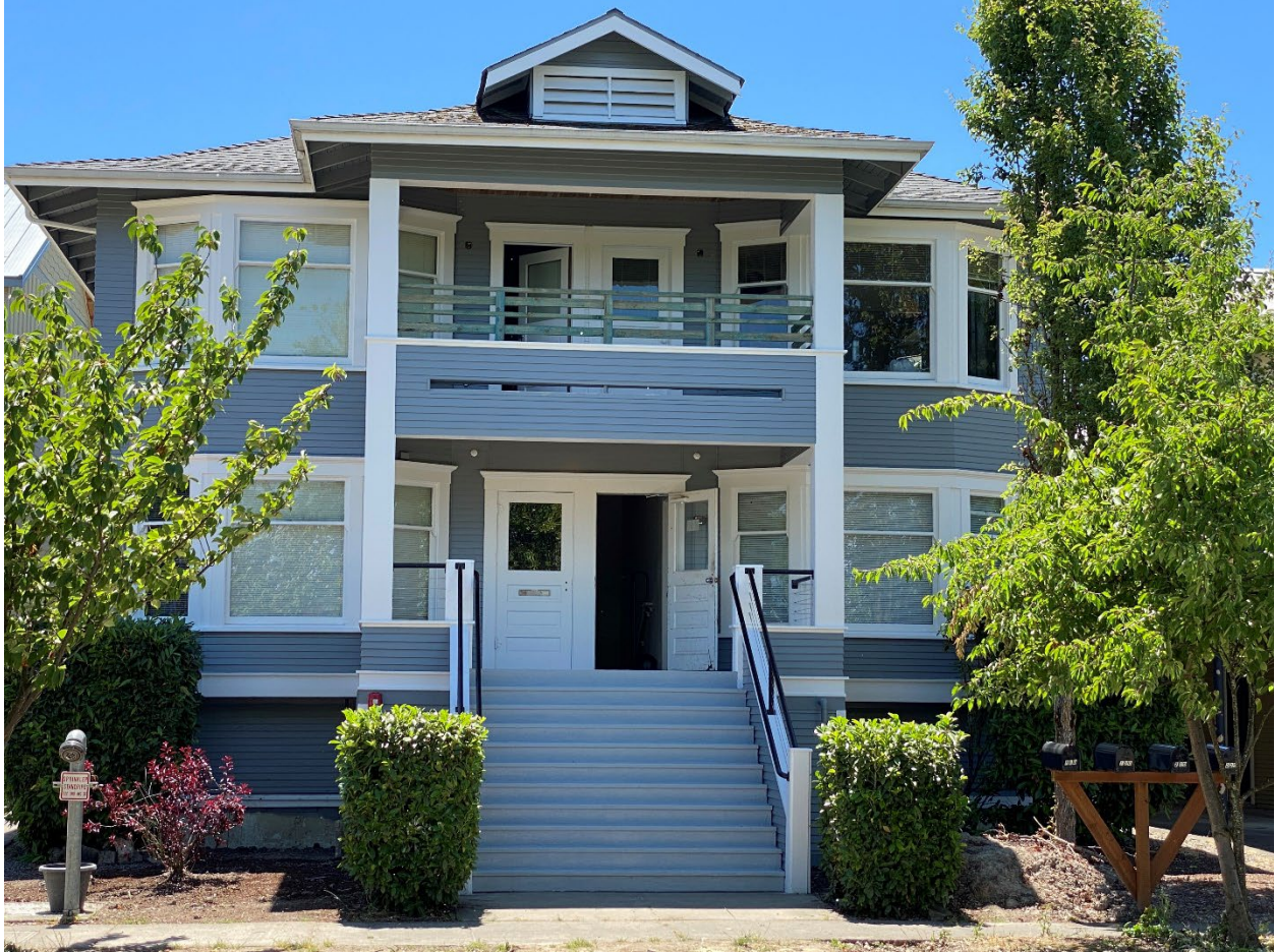
Figure 4: North Elevation, July 2024
