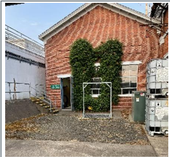
Photo 2 Vine Street – Raw Water Pump Station Exterior
