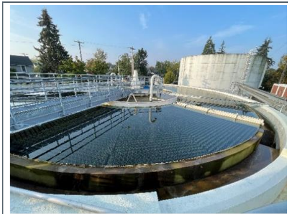
Photo 8 Vine Street - Concrete Accelerator 1
