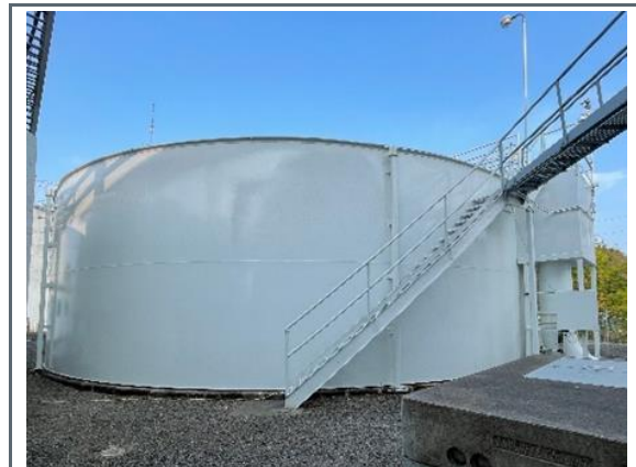
Photo 9 Vine Street - Steel Accelerator 2
