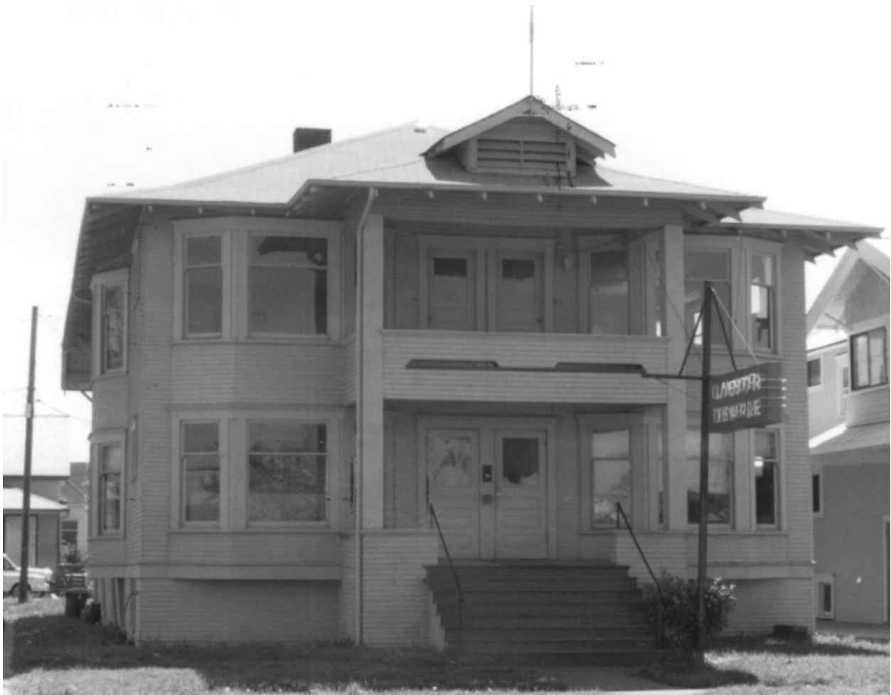
Figure 1: North Elevation, Historic Resource Form
