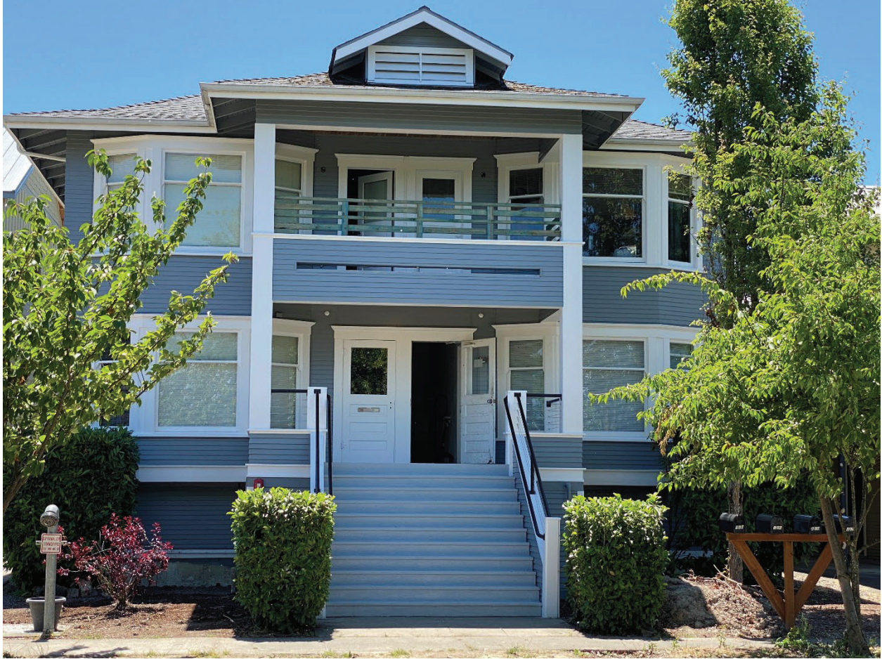
Figure 4: North Elevation, July 2024
