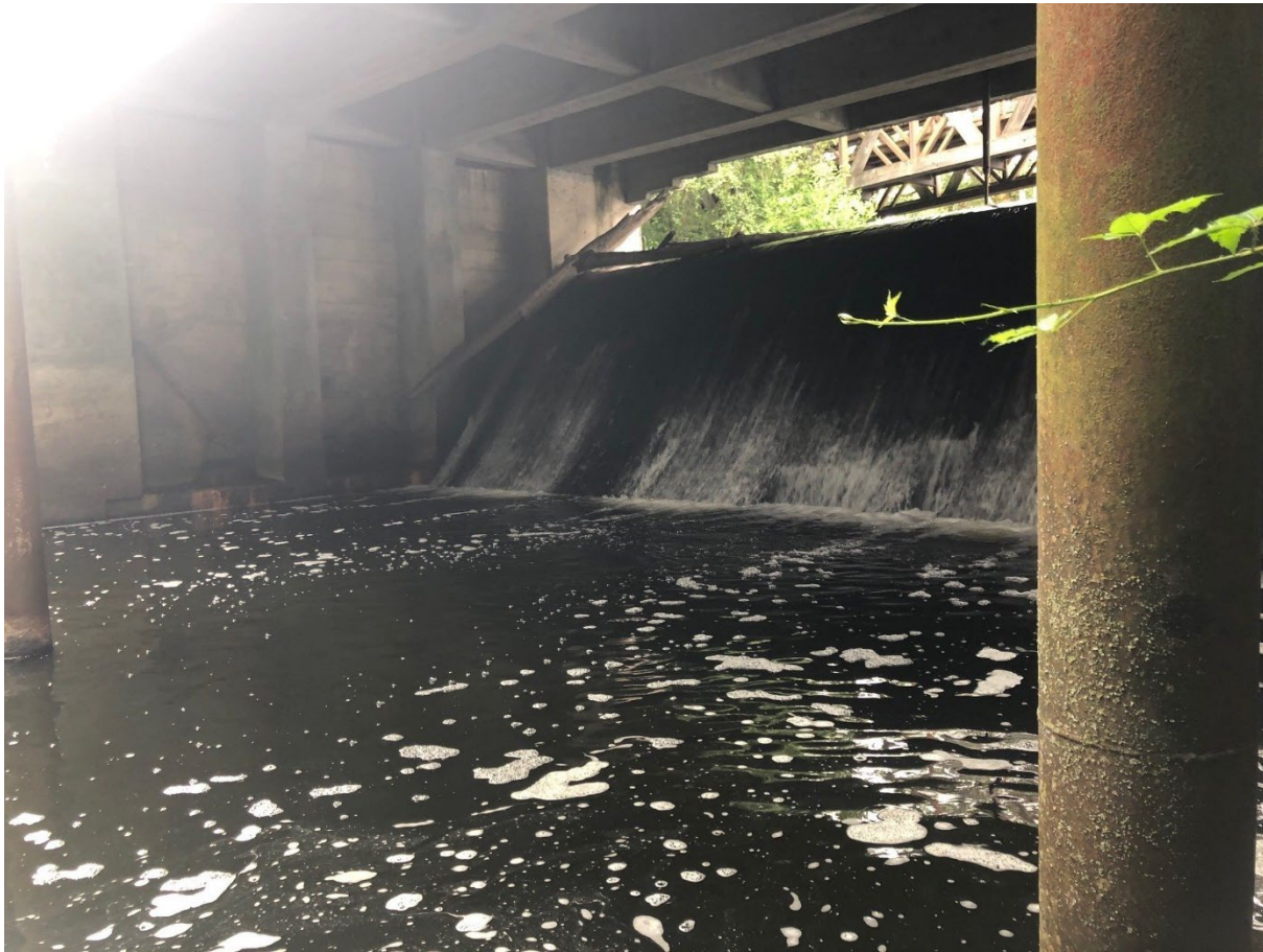
Figure 7. Spillway under low flow conditions (showing backwater conditions).
