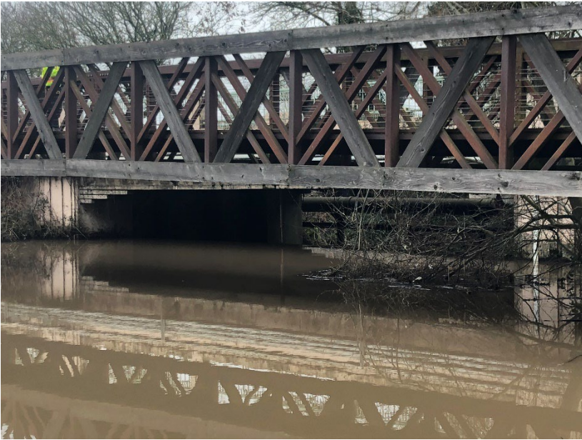
Photo 9: Upstream face of spillway
