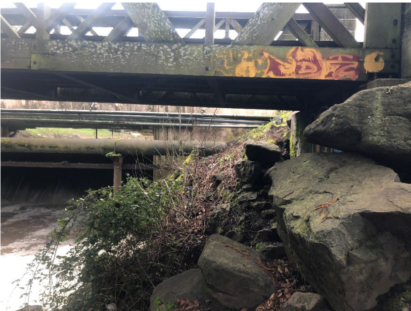
Photo 7: Left abutment of downstream pedestrian bridge
