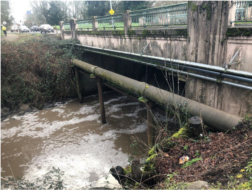
Photo 5: Downstream face of spillway bridge
