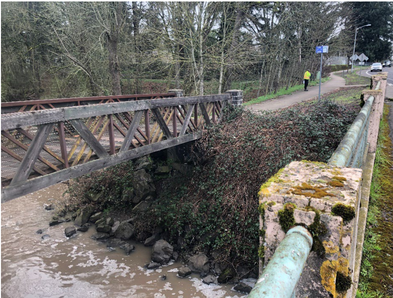
Photo 3: Looking towards right bank between spillway bridge and downstream pedestrian bridge
