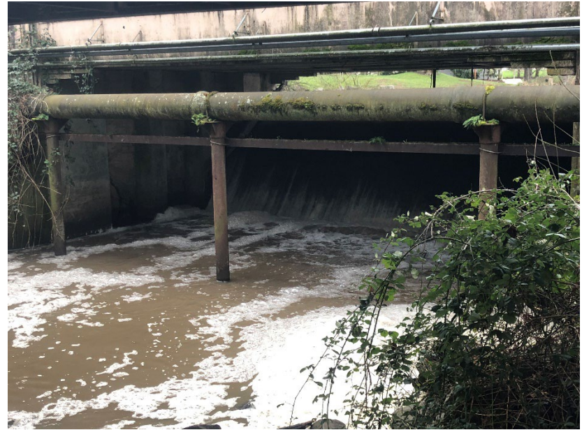
Photo 6: Looking upstream to spillway
