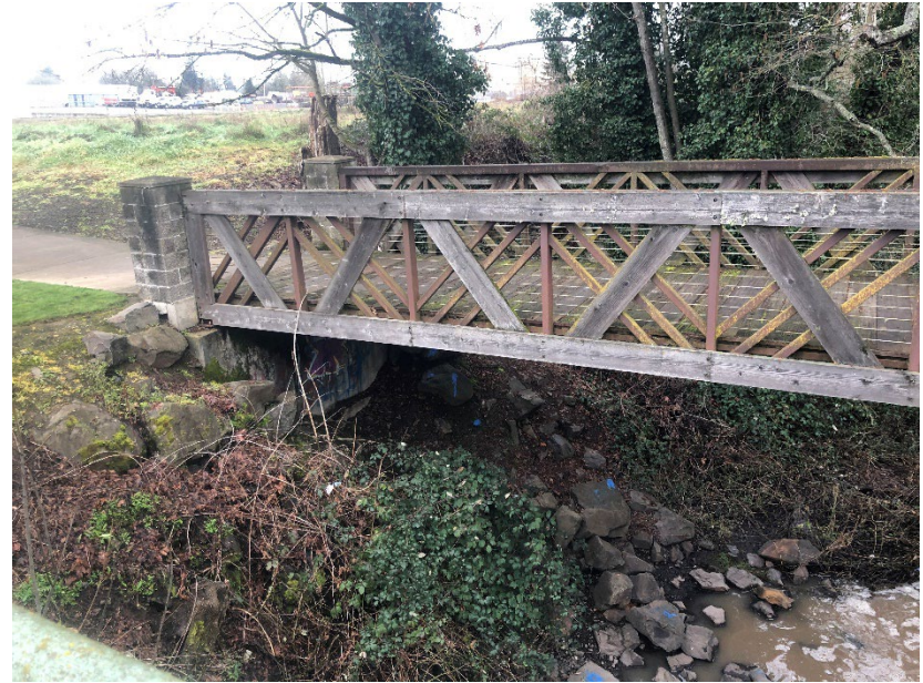
Photo 2: Looking towards left bank between spillway bridge and downstream pedestrian bridge
