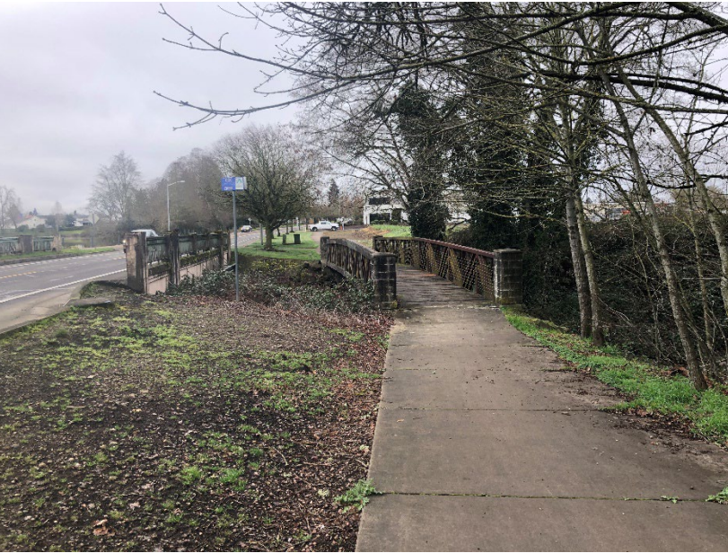
Photo 1: Looking right to left (west) along downstream pedestrian bridge
