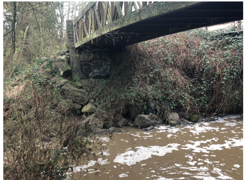
Photo 8: Right abutment of downstream pedestrian bridge
