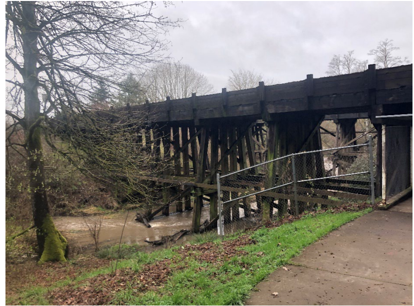
Photo 10: Upstream face of RR trestle bridge
