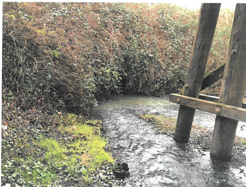
Inlet of P&W Culvert (1 – 12.00' dia. Corrugated Metal Pipe)
