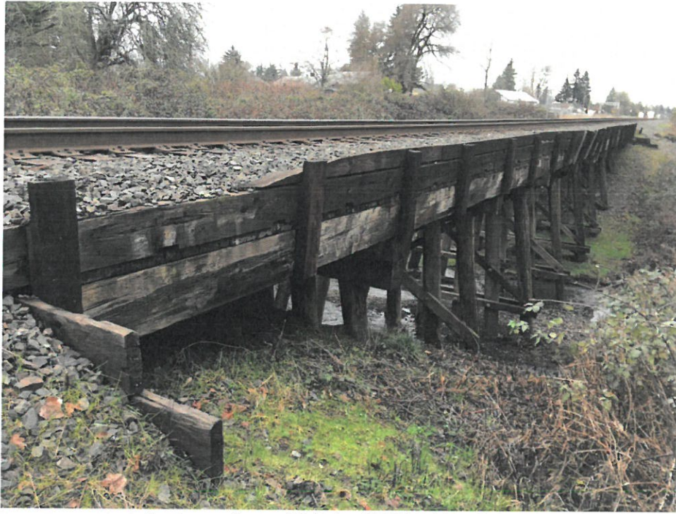
Upstream Face of Existing UPRR Bridge 691.77
