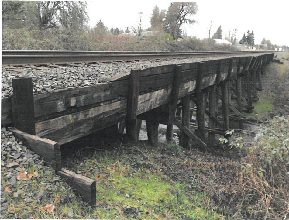
Upstream Face of Existing UPRR Bridge 691.77
